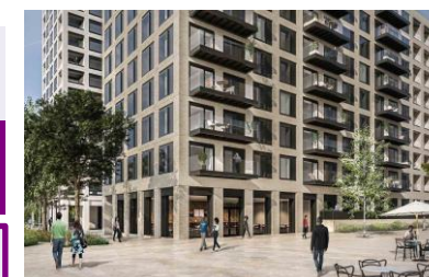
Deanston Wharf, UK
