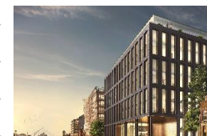
Dublin Landings, Ireland
