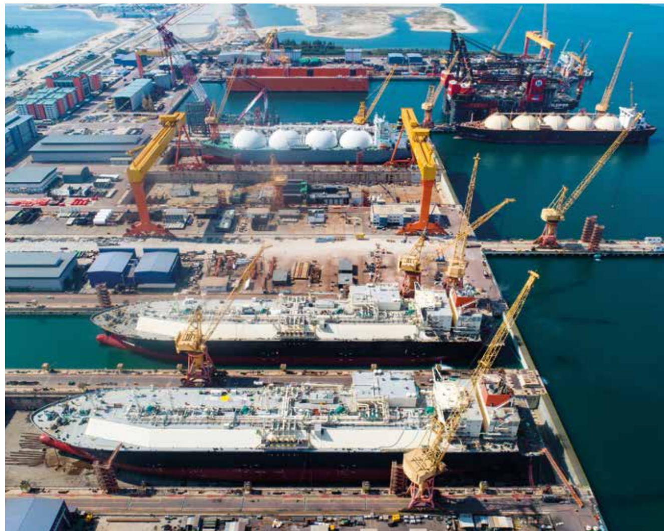
The Tuas Boulevard Yard strengthens Sembcorp Marine's value proposition as a one-stop solutions provider offering optimal production efficiency, cost-effective execution and shorter project delivery times
