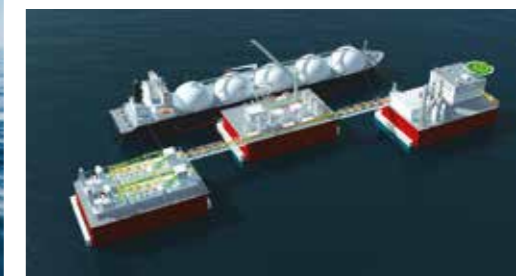
Gravifloat: Modularised liquefied natural gas and liquefied petroleum gas terminals
