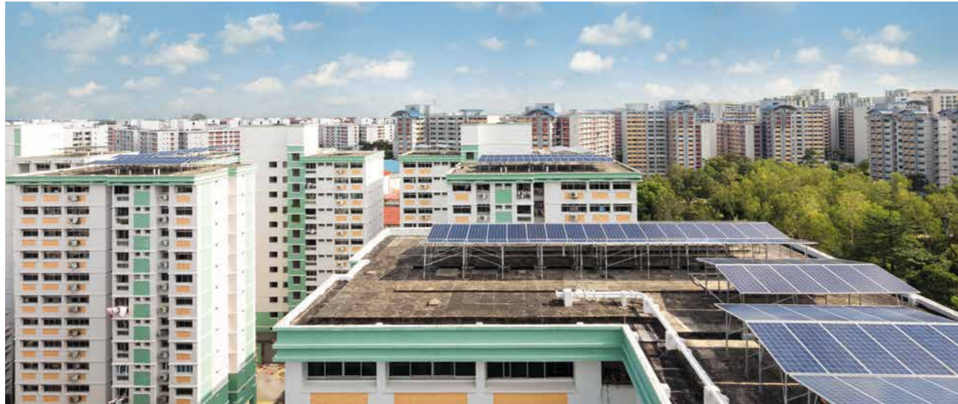
Sembcorp's solar power business in Singapore is growing well, with rooftop assets that generate renewable energy for the land-scarce city state
