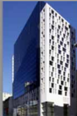
77 King Street Office Tower, Sydney
