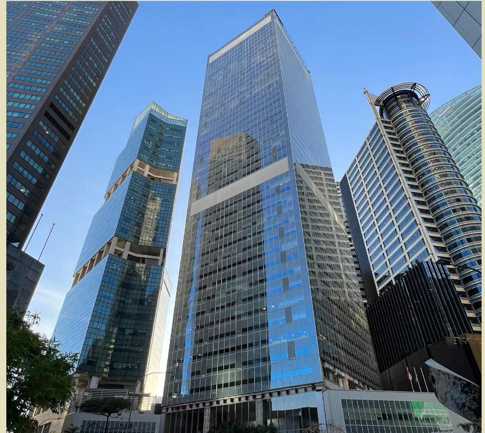
A low-emissivity double glazing curtain wall system is a key feature in Singapore Land Tower's AEI and helps to reduce heat transfer.
