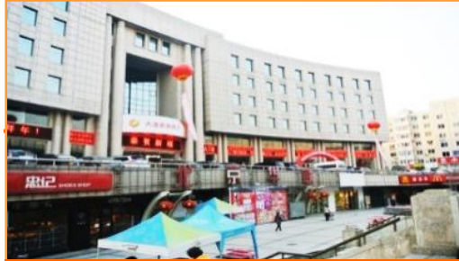
Dalian Jinsanjiao Property
