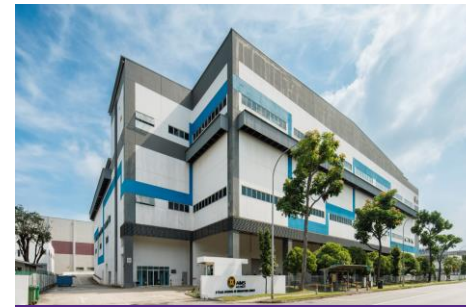
8 Tuas Avenue 20, Singapore
