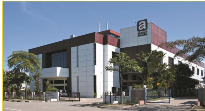
26 Tuas Avenue 7, Singapore
