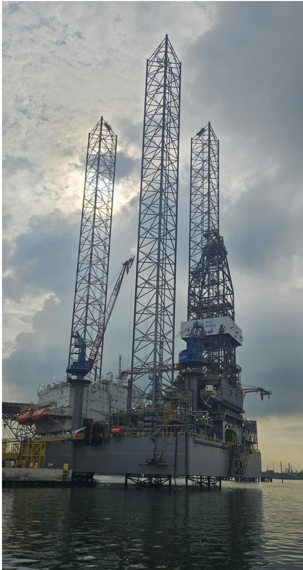
Caption: Built to the KFELS Super B Class rig design, the Jackup rig, Var can also accommodate up to 150 persons with full amenities.
