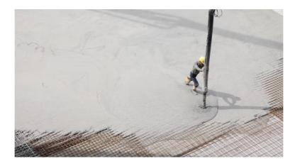
With PanU NewGen SCC, only one worker is required to guide the concrete pumping pipe around the slab area. Regular concrete will require several workers to work closely together to manually vibrate and compact the material into place.
