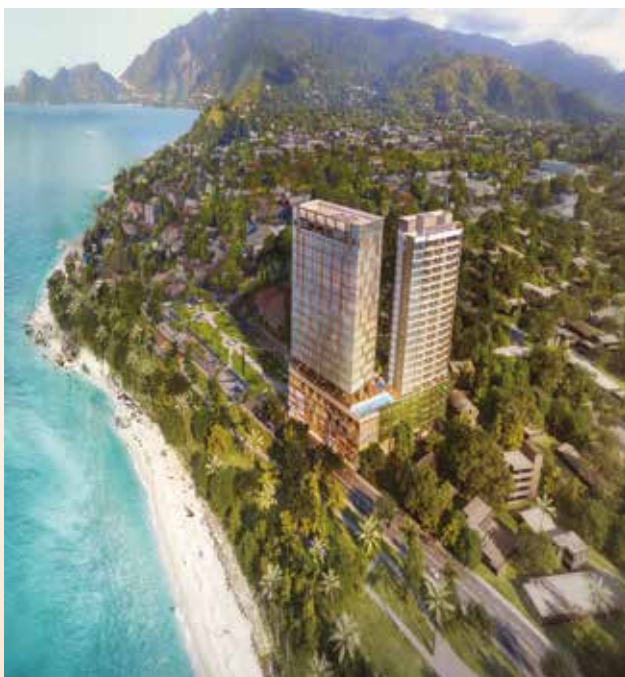
Actual aerial view of vicinity of Timor Marina Square
