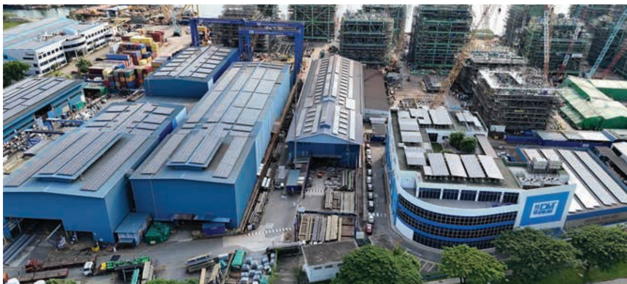
DM's building rooftop installed with solar panels
