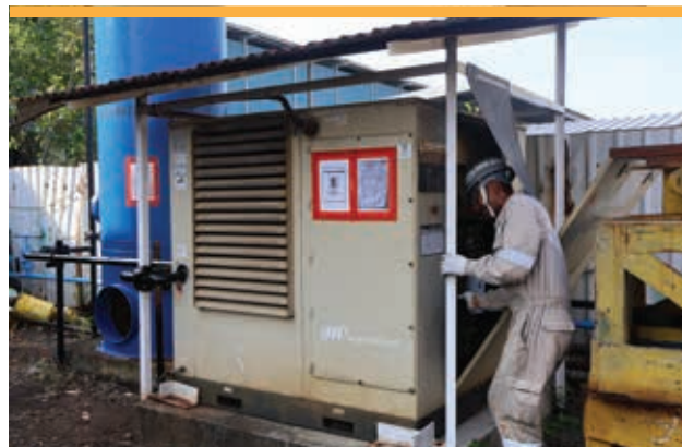
Worker maintaining electric air compressor.
