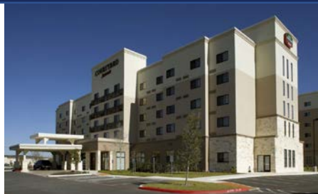
Courtyard San Antonio at The Rim
