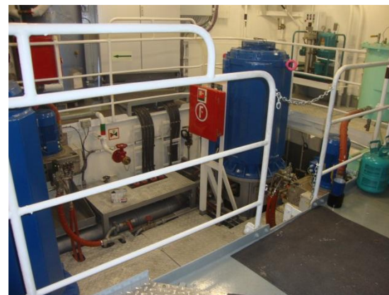
Forward thruster room
