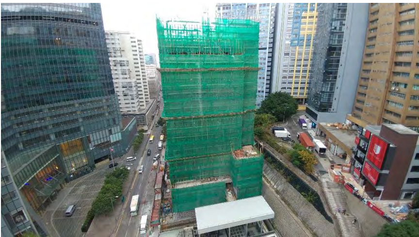
Existing site undergoing construction
