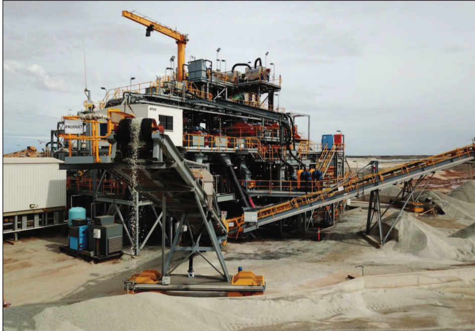
Figure 20: Stage 1 DMS plant
