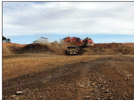
Mining excavations to provide additional sump capacity
