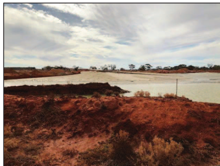
Tailings discharge into Boreline Pit
