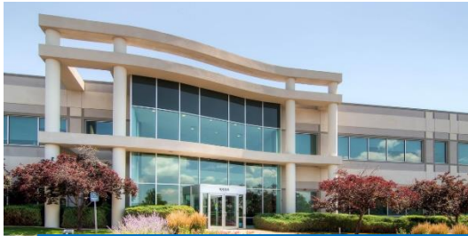
Westmoor Center, Denver
