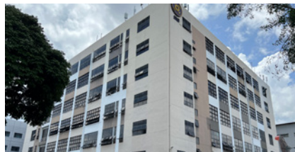
19 61 Yishun Industrial Park A
