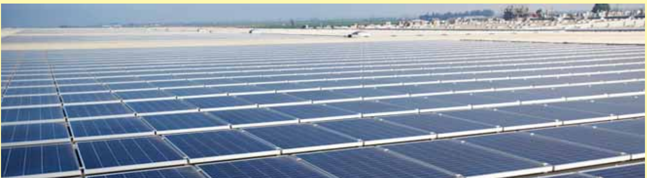
Solar panels in Hanford facility in California, USA
