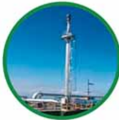
Waste-To-Energy Biogas Plant
