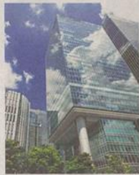
GIC is taking up the entire office component of Pacific Century Place Marunouchi, next to Tokyo Station
