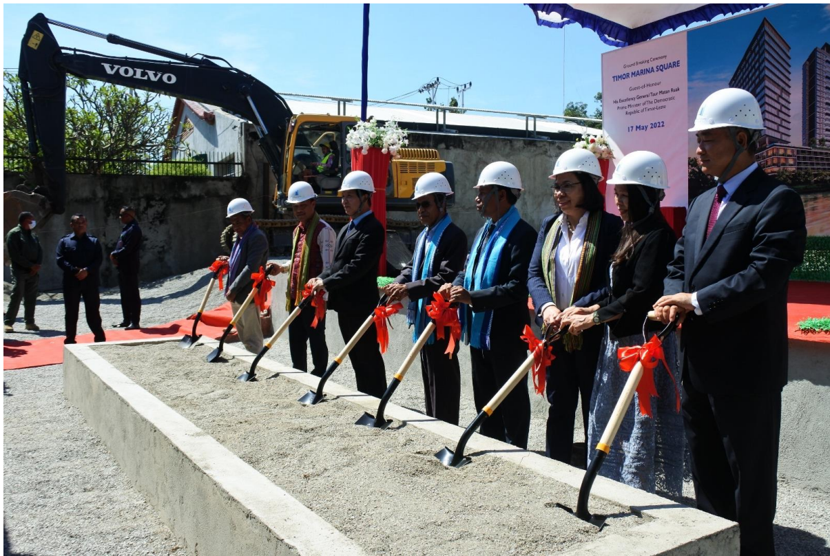
Groundbreaking ceremony performed by Directors of the consortium and ministers led by the Prime Minister of Timor-Leste.
