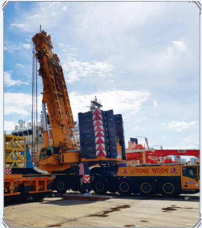
Location: Pandan Loop, Singapore Equipment: 500 Ton Mobile Crane Scope of Work: Heavy Lifting Services
