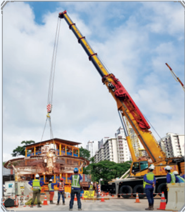
Location: Lower Delta, Singapore Equipment: 500 Ton Mobile Crane Scope of Work: Heavy Lifting Services
