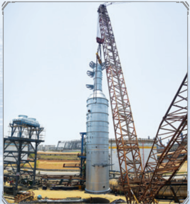
Location: Mumbai, India Equipment: 1250 Ton Crawler Crane Scope of Work: Heavy Lifting Services
