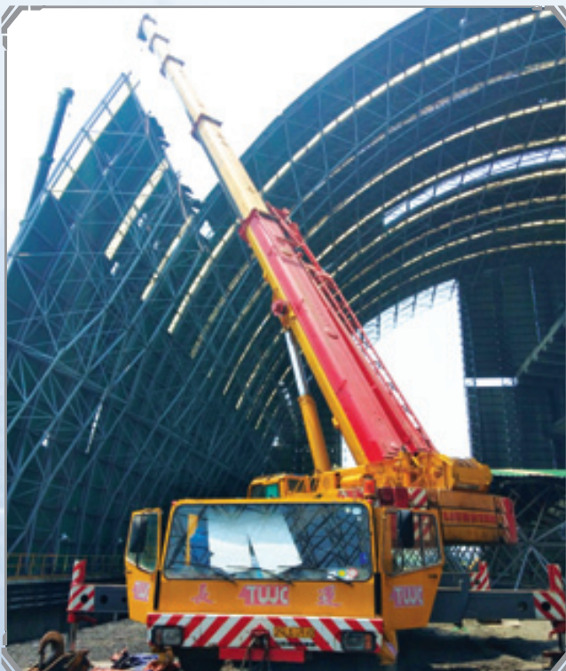
Location: Ha Tinh, Vietnam Equipment: 160 Ton Mobile Crane Scope of Work: Heavy Lifting Services
