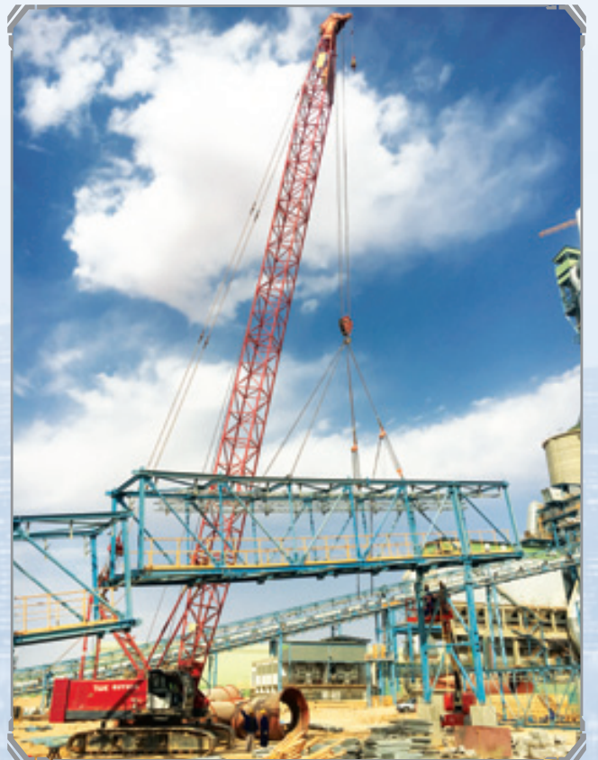
Location: Al Kharj, Saudi Arabia Equipment: 50/55/80/120/200/280 Ton Crawler Cranes, 100 Ton Mobile Crane, 70 Ton Rough Terrain Crane Scope of Work: Equipment Rental
