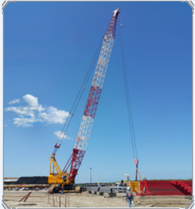
Location: Bang Pakong, Thailand Equipment: 150 Ton Crawler Crane, 45 Ton Rough Terrain Crane Scope of Work: Equipment Rental
