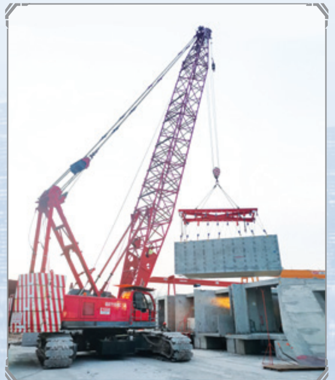
Location: Johor, Malaysia Equipment: 150 Ton Crawler Crane Scope of Work: Equipment Rental
