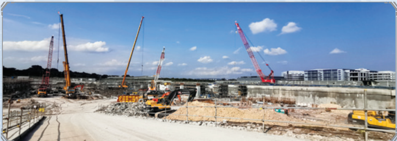
Location: Jalan Bahar, Singapore Equipment: 100 Ton Crawler Crane, 200 Ton Mobile Crane Scope of Work: Heavy Lifting Services
