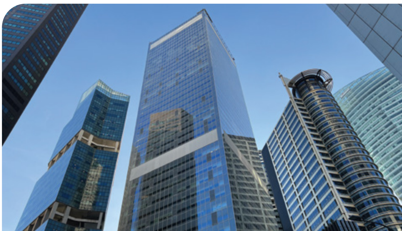
Singapore Land Tower's asset enhancement initiative achieved several key milestones in 2023, including the completed installation of the new facade.
