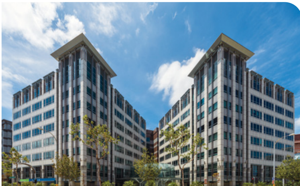
With the Green Mark Platinum certification of Tampines Plaza 1 & 2 in 2023, all nine Singapore commercial properties are Green Mark certified.
