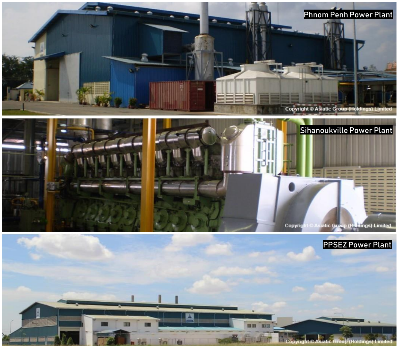
Figure 2. Colben Energy’s three operational power plants in Cambodia
