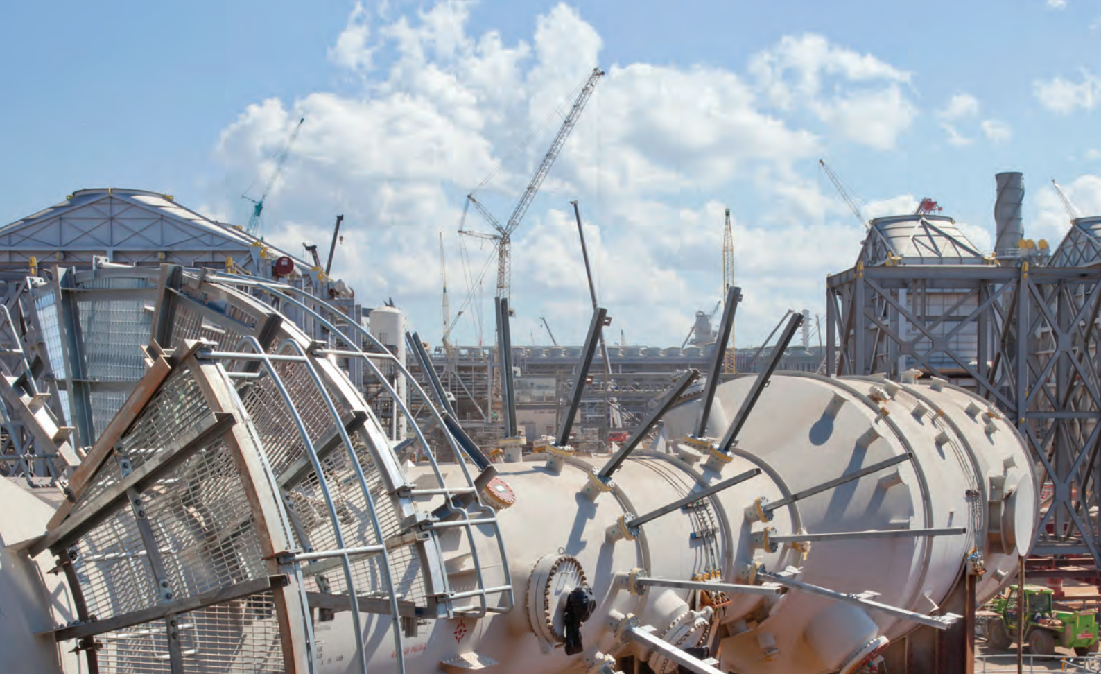
JKC - INPEX-operated Ichthys Project Onshore LNG Facilities, Bladin Point, Northern Territory
