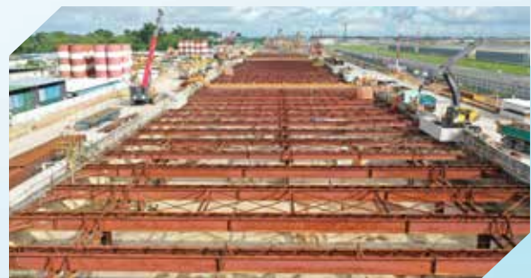
Project Photo - Roof Top with Temporary Struts
