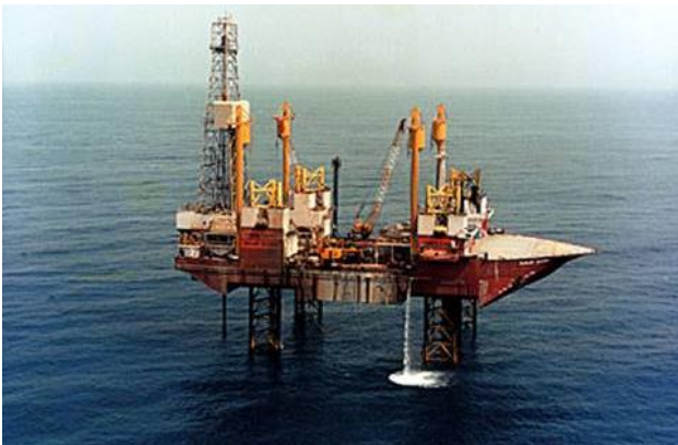
Sagar Samrat MODU being converted to MOPU
