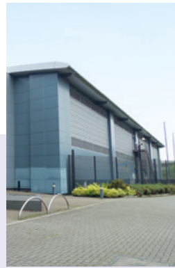
Cardiff Data Centre
