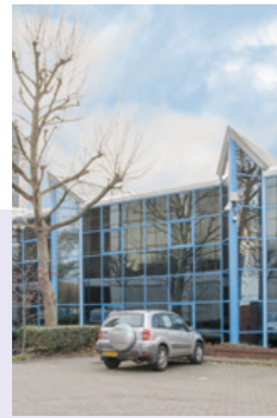
GV7 Data Centre
