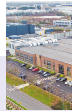
Keppel DC Dublin 2
