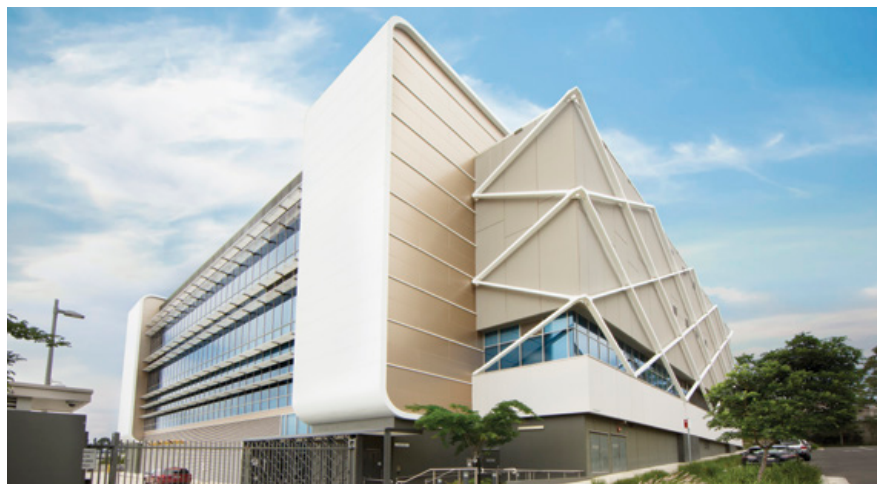
Gore Hill Data Centre is located within the Gore Hill Technology Park in Sydney, Australia.
