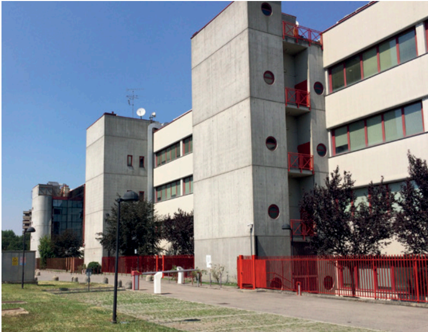
Milan Data Centre is located approximately 8km away from Milan's city centre.
