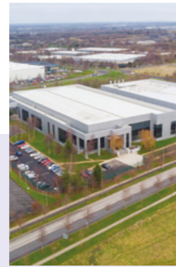
Keppel DC Dublin 1
