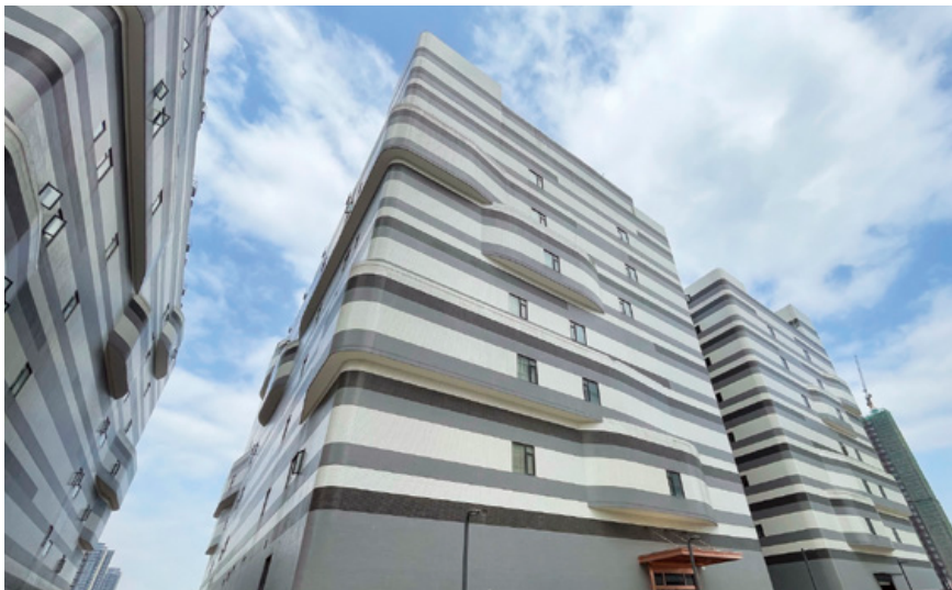
Guangdong Data Centre is located in the Bluesea Intelligence Valley Mega Data Centre Campus in Jiangmen, Guangdong Province in China.
