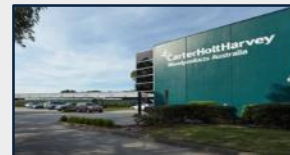
24 41 – 45 Hydrive Close, Dandenong South
