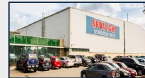
19 217 – 225 Boundary Road, Laverton North
