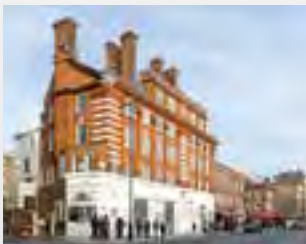
Former Westminster Fire Station, United Kingdom
