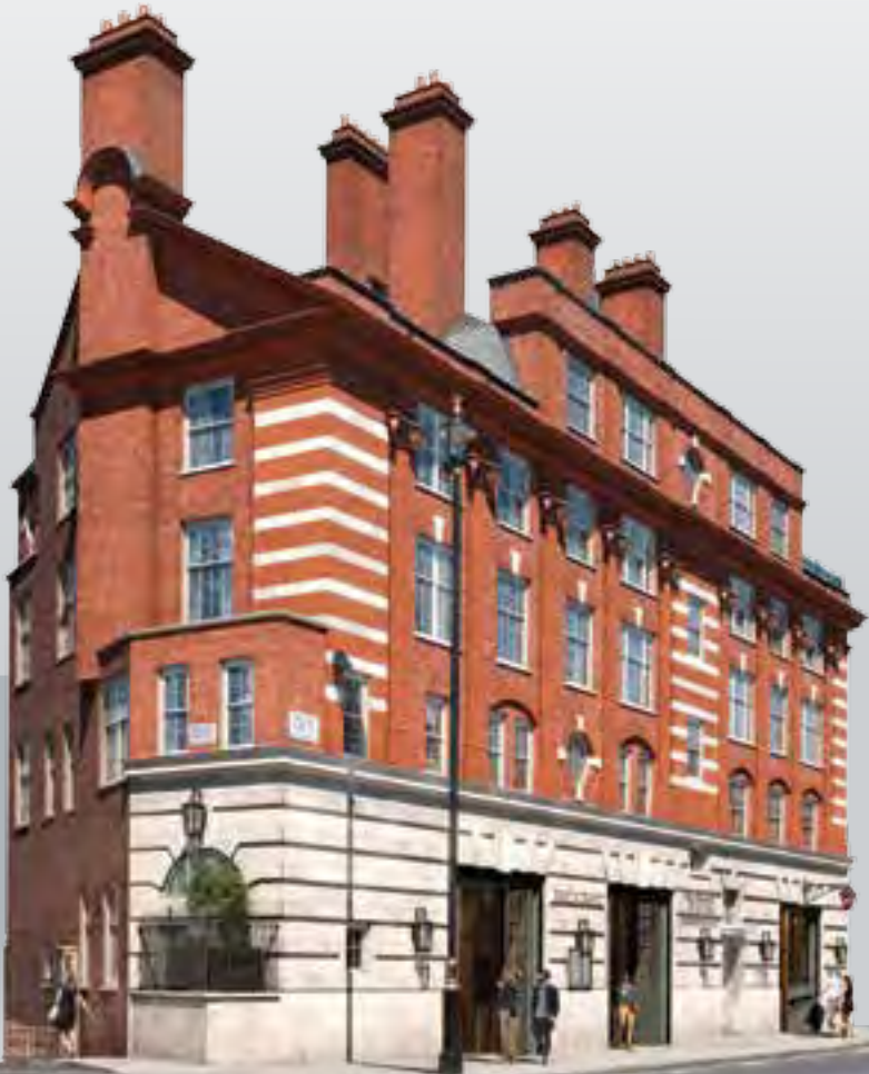
Former Westminster Fire Station, United Kingdom 3
