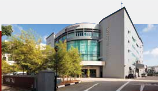
25 Changi South Avenue 2 2
