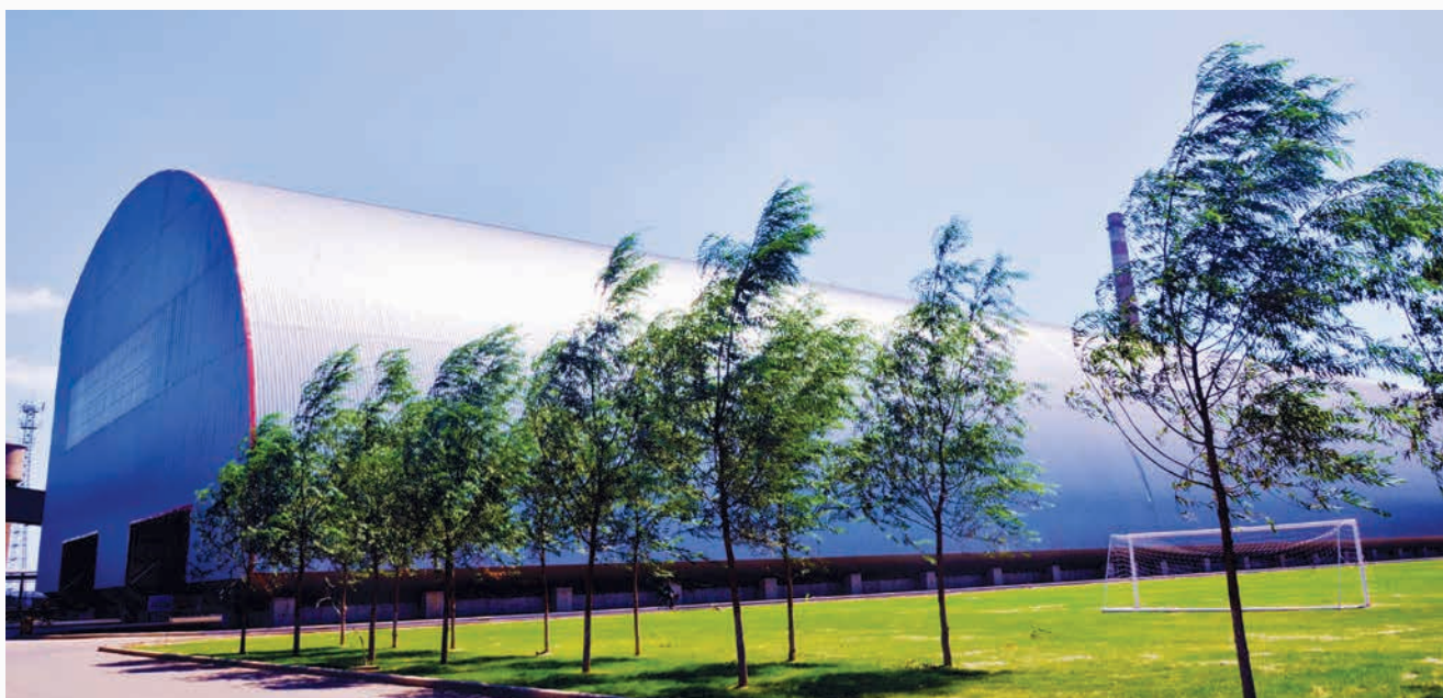
Enclosed raw materials warehouse to keep the amount of dust to a minimum.
