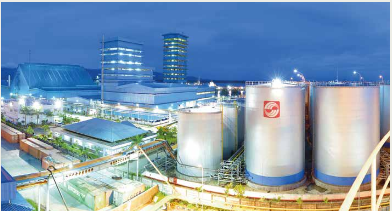
Our refinery and facilities in South Kalimantan where our processed products are produced.
