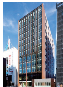
Kichijoji Fukoku Seimei Building completed in fiscal 2023.
