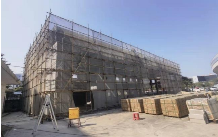
Construction photo of TCA Guangzhou Genesis
