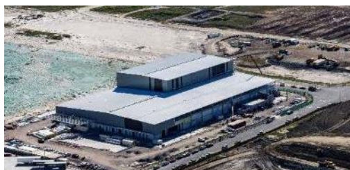
Corner Heron Drive and Curlew Street, Port of Brisbane, QLD (under construction)
