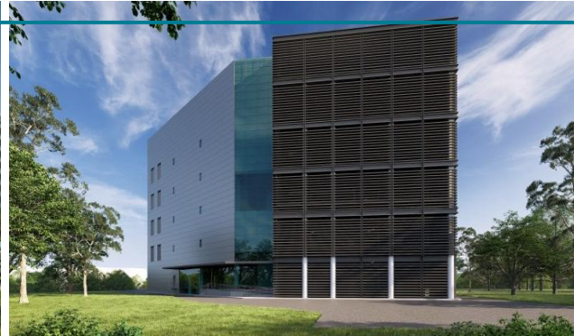
Taiwan Data Centre Campus
