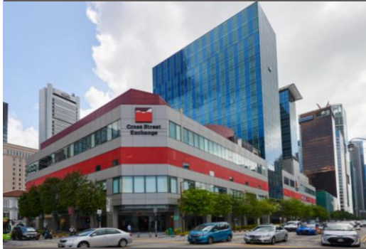
Cross Street Exchange
