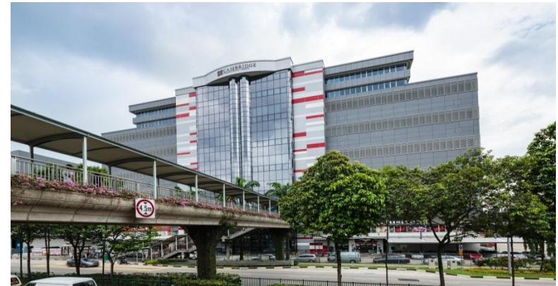
30 Toh Guan Road (Annex Block)
