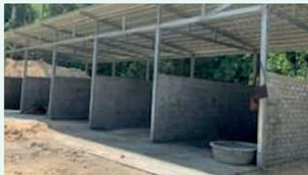
The final waste segregation and recycling area constructed from the hand made bricks
