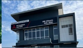
Mitsubishi Motors 3S Dealership Bandar Bukit Raja
