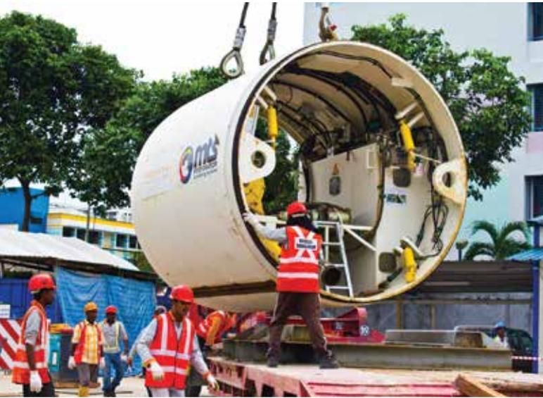
TBM (Tunnel Boring Machine) Launch at Nee Soon (MH14) (Sewerage Scheme to Phase Out Nee Soon Pumping Station – Contract 1)
