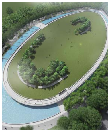
▲ Marina East Desalination Plant
