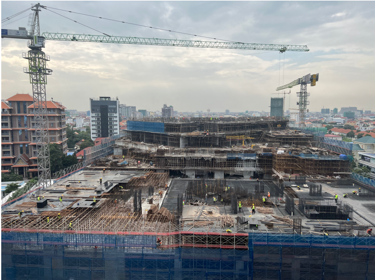
(Main Construction Site for Royal Platinum mixed-use project)
