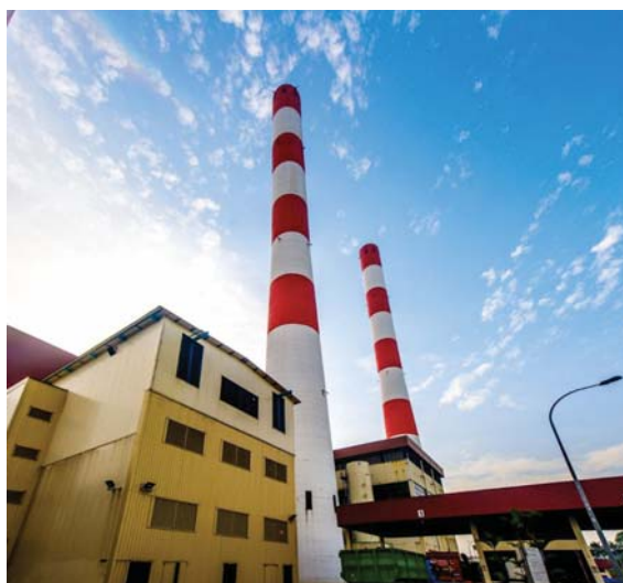
Senoko WTE plant, Singapore
