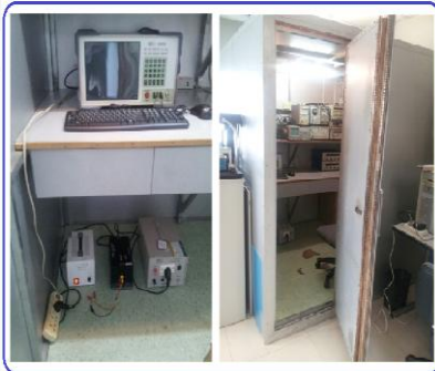
EMI Testing Equipment
