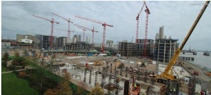
Construction progress as at 15 Oct 2015
