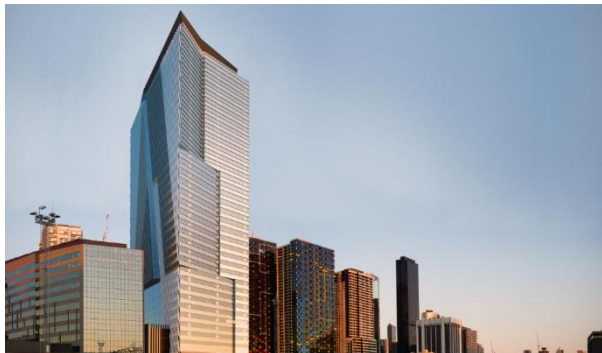
Topped out 311 Spencer Street in Melbourne
