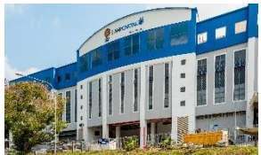
11 Changi South St 3
