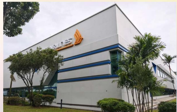
SBO facade with cool paint
