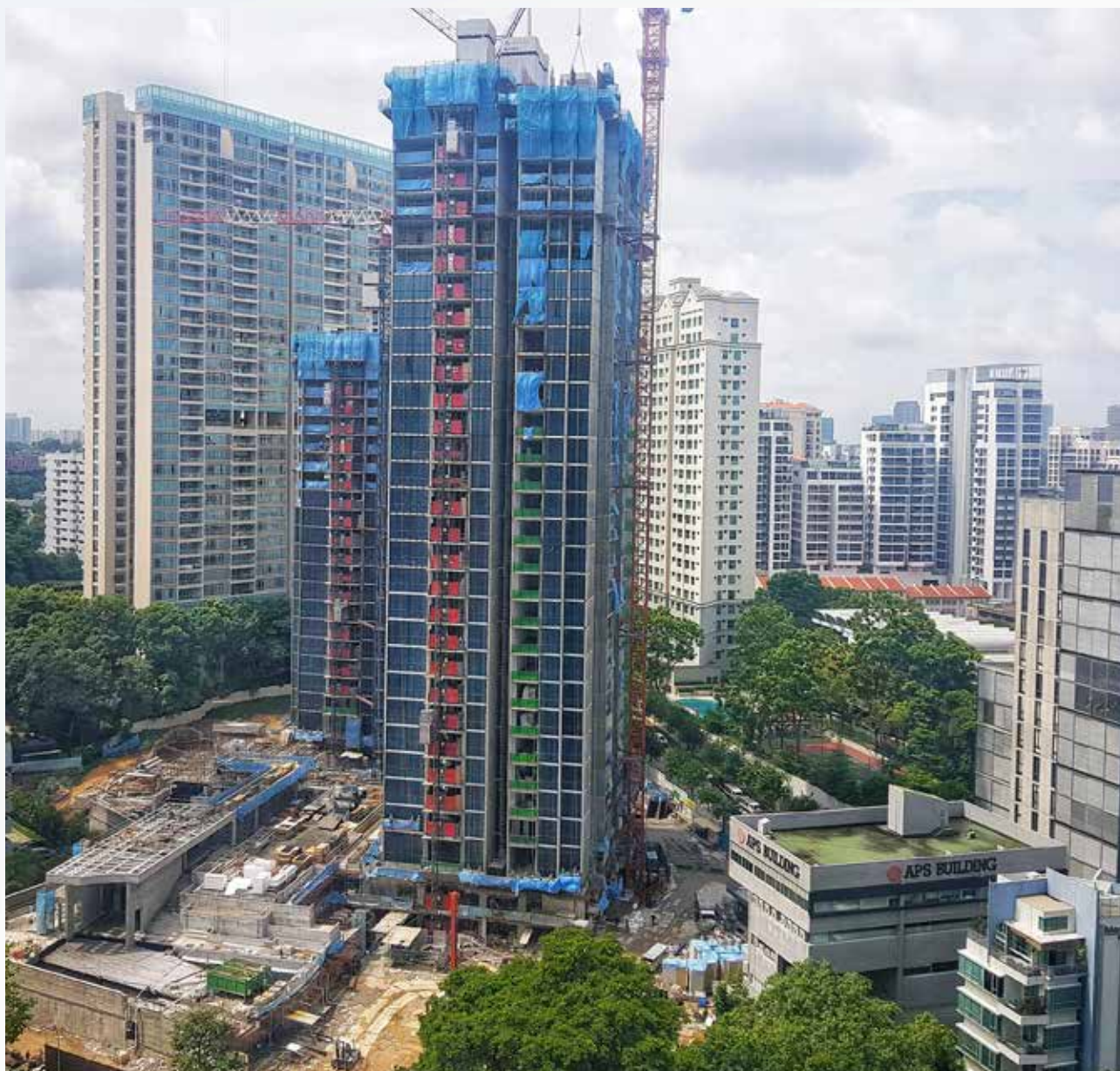
▲ Ongoing project – Martin Modern
