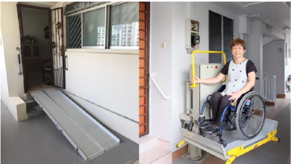
Portable ramp (left) and wheelchair lifter to help residents access their flats more easily and safely. (Photos: Housing & Development Board)
